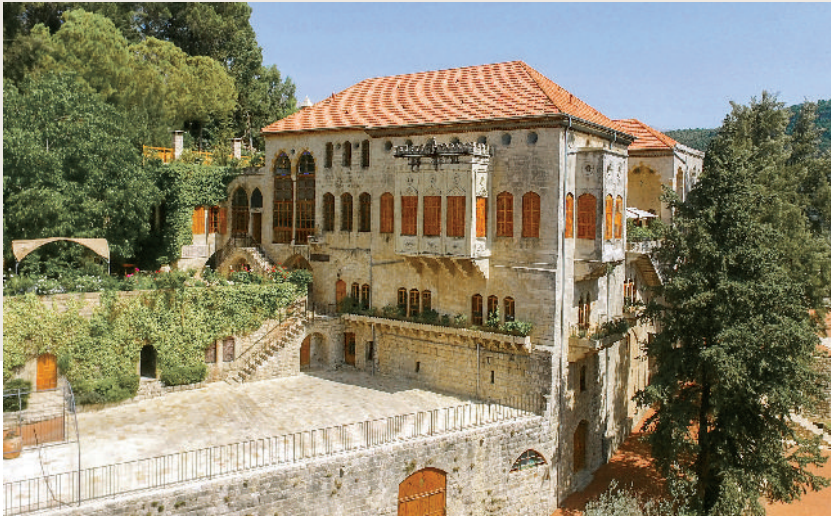
The north and west facades of the first building
