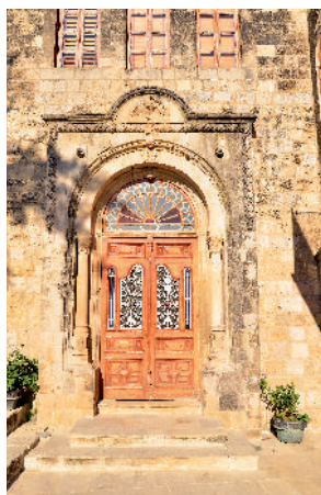
Entrance to the main building, modified during the twentieth century
