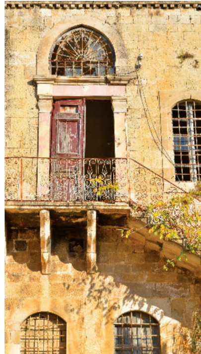
Entrance to the first floor
