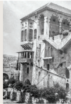
The First Building, around 1930
